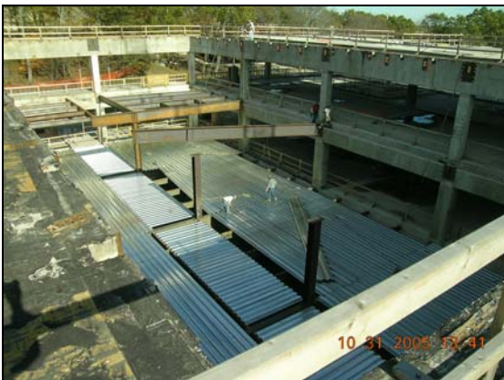
This project included the abatement and demolition of old office and industrial facades and all interior building systems down to the basic structural frames on three existing headquarters campus buildings as part of the ‘Base Building Scope’ or renovation work and not as a property preparation pre-development step; some new in-fill and adding a new top floor proceeded installation of all new building systems and curtain wall / window facades.
