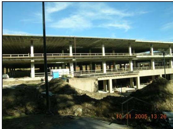
This project included the abatement and demolition of old office and industrial facades and all interior building systems down to the basic structural frames on three existing headquarters campus buildings as part of the ‘Base Building Scope’ or renovation work and not as a property preparation pre-development step; some new in-fill and adding a new top floor proceeded installation of all new building systems and curtain wall / window facades.
