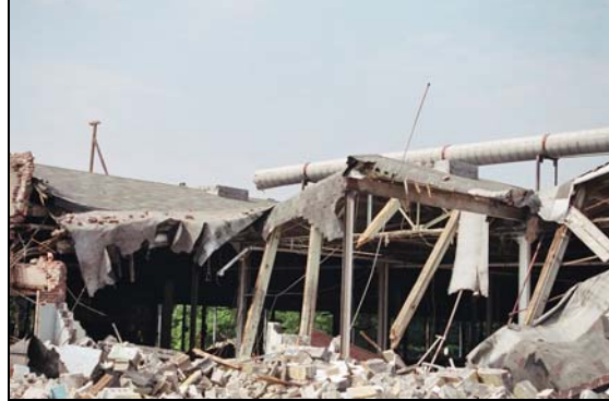
Building demolition can include prior environmental abatement and an extensive range of old structural systems and materials; demolition requires experienced demo contractors and strict safety standards and procedures
