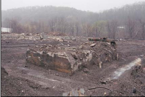
Many of the multifamily projects we have been involved with Are redeveloping ‘Brownfield’ property containing old industrial Buildings requiring site preparation by the developer; view Above shows old concrete foundations uncovered during Demolition – many were larger and deeper than expected
