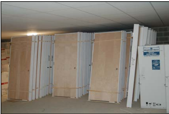
On-site Stored Materials – Doors + Frames, well organized, properly stacked and supported and stored under cover well protected from weather and vandal exposure
