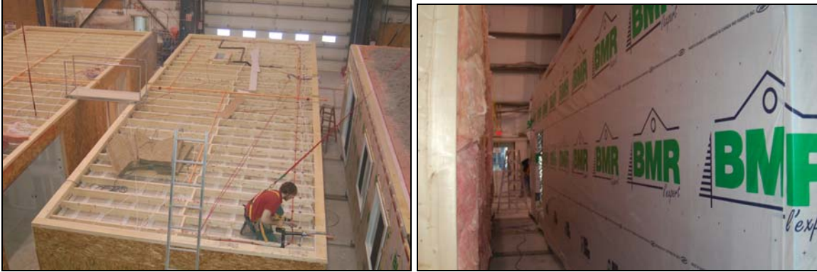
View of modular housing construction using assembly line techniques to fabricate each 'box'; each station along the assembly line uses workmen trained in each step of the fabrication and also uses 'just-in-time' materials and building components to supply the production line. The construction work takes place within a large 'heated and weather protected' building. After each box is completed it is wrapped in weather protecting plastic sheets and moved into temporary storage in the factory yard.
