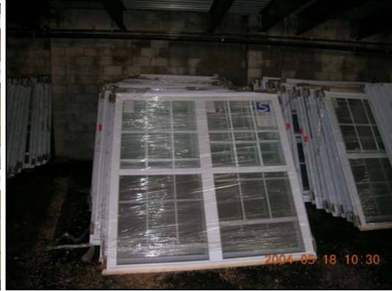
On-site Stored Materials – windows stored under cover but inadequately protected and stacked, racking of frames is judged to be highly likely by time of installation, storage methods and interior environmental condition was found to not meet Manufacturers requirements – payment was not approved.
