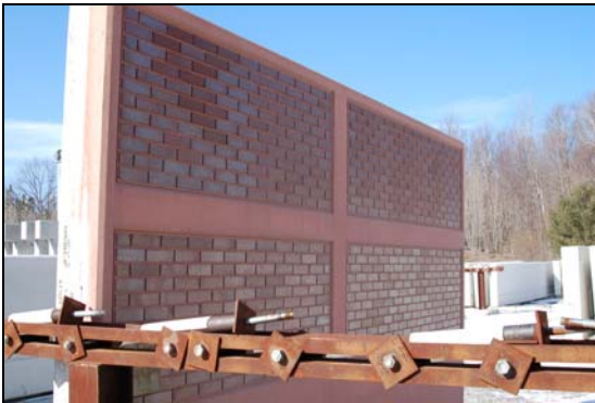
Off-site stored Materials – Architectural Precast Concrete + Face brick panel ready for shipment and erection, however, Construction at site is not ready for erection phases
