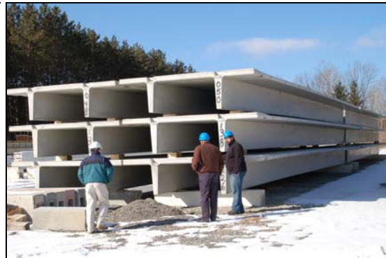
Off-site Stored Structural Precast Concrete Garage Floor ‘Twin-tee’s’ stock-piped at plant yard ready for shipment and erection
