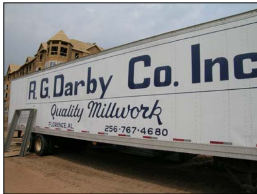
On-site Stored Materials – generic non-fabricated millwork running trim stock stored in subcontractor’s trailer parked on construction site – how easy is it to take trailer off-site?
