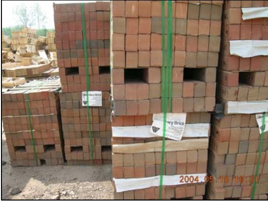
On-site Stored Materials – brick in the foreground, fabricated Wood trusses for multi-family housing project; brick is Generic – floor trusses are a more unique product for this specific project, total supply of both materials will not be installed within next (30) days of construction.
